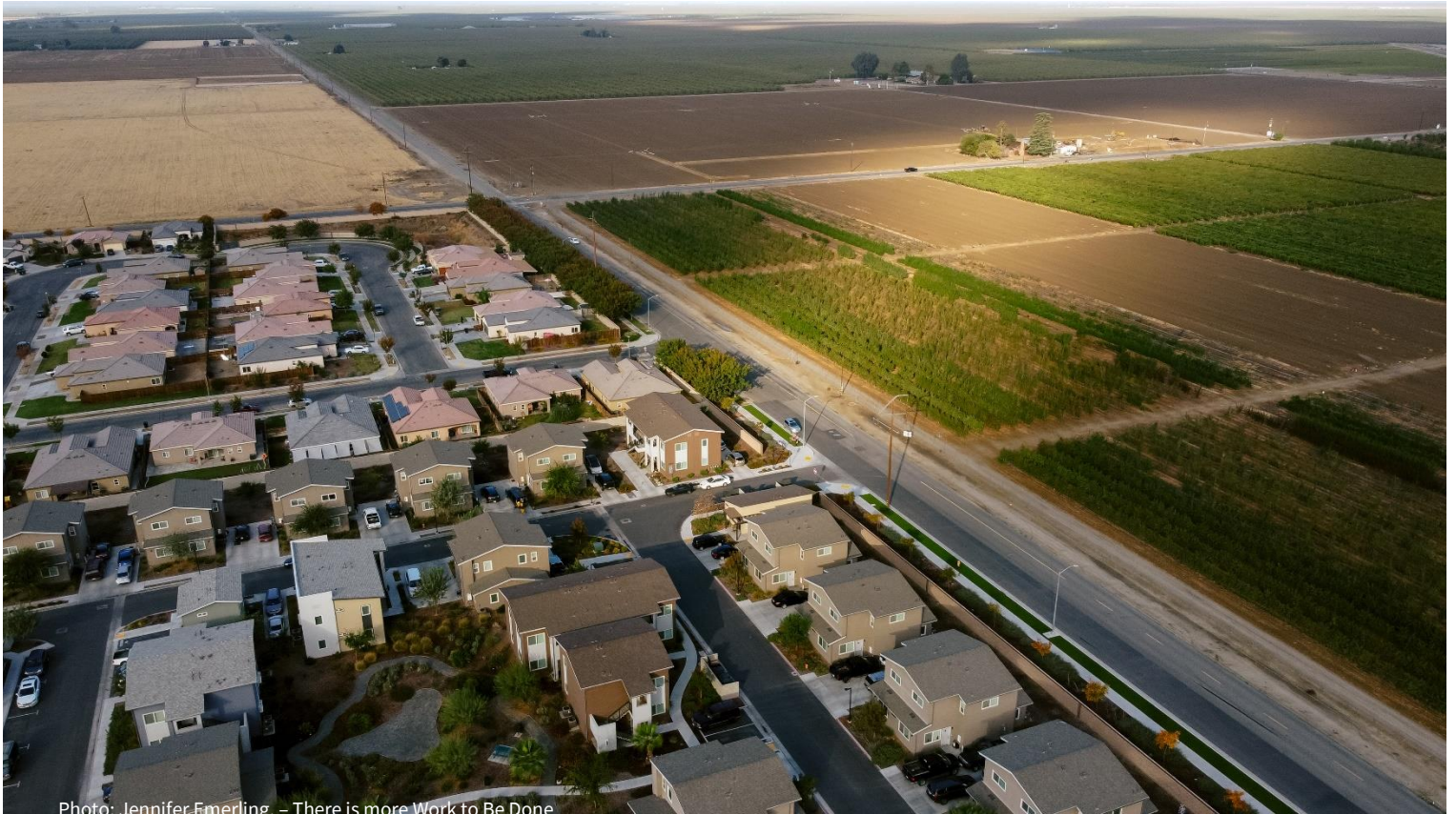
Photo: Jennifer Emerling – There is more Work to Be Done
